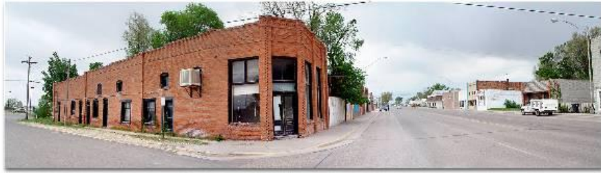
ESTANCIA, NM Hwy 41 0/10/04 2:30 LOOKING SOUTH
